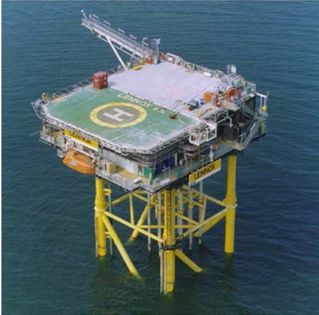
Figure 2-4: Lennox (LD) Platform Overview
